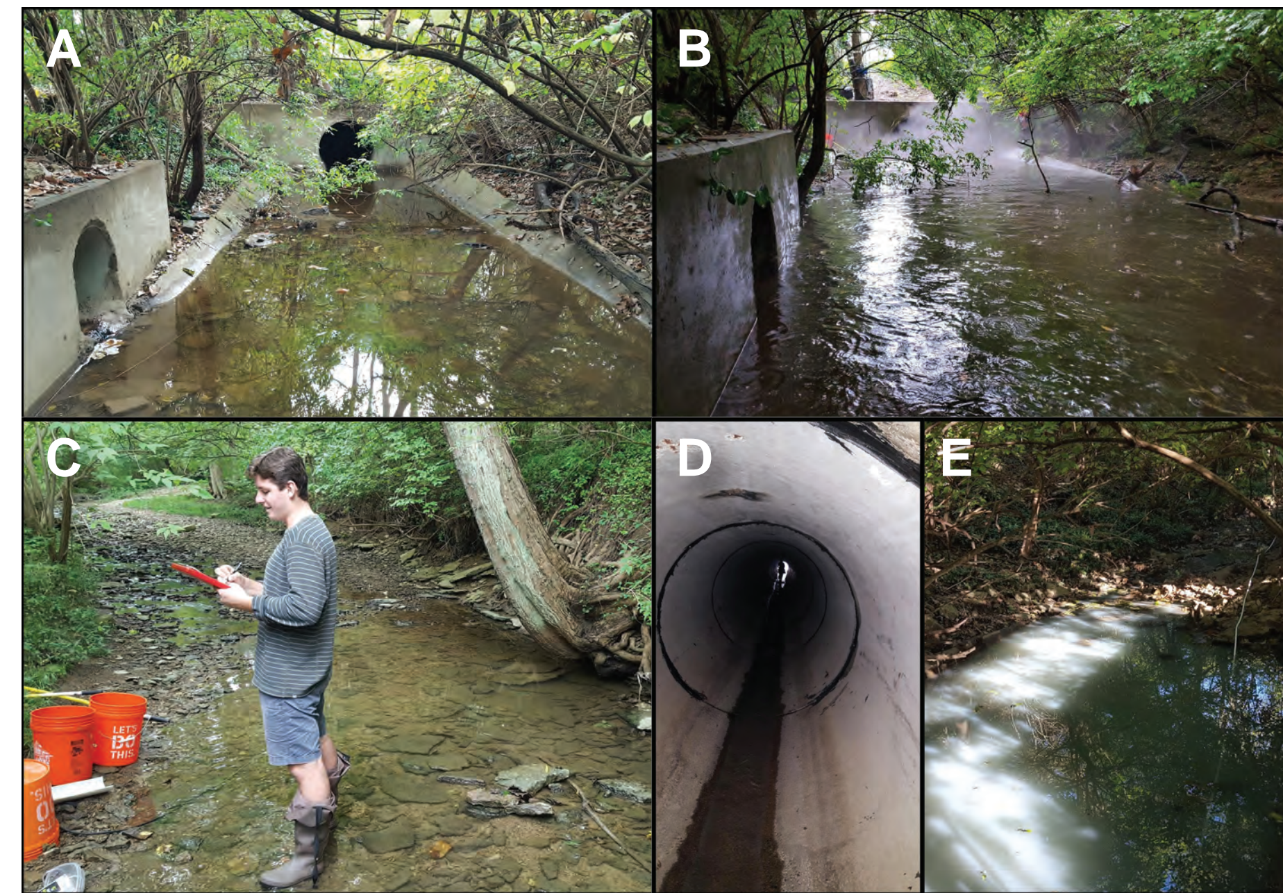
▲ Figure 2. In urban settings, streams are often buried or culverted and in addition to hydrologic modification, are impacted by a variety of human impacts. A) Headwaters of Cooper Creek, a tributary to Mill Creek in Cincinnati, OH. A stormwater drainage network is the primary source of flow. B) Flows increase rapidly following storms—flows shown are about 15 minutes after a moderate, localized thunderstorm, which increased flows dramatically. C) High flows and frequent erosion events lead to channel overwidening or incision. In addition, pipes buried under streams (e.g., sanitary sewers) can capture surface flows, dewatering the creek or leak contaminants into the channel. D) Although culverts are simple habitats, they may provide overhead cover and pool habitat that is otherwise scarce. E) Non-point sources of pollution, as well as illicit dumping (e.g., dumped paint from an autobody shop shown here) directly impact urban water quality
